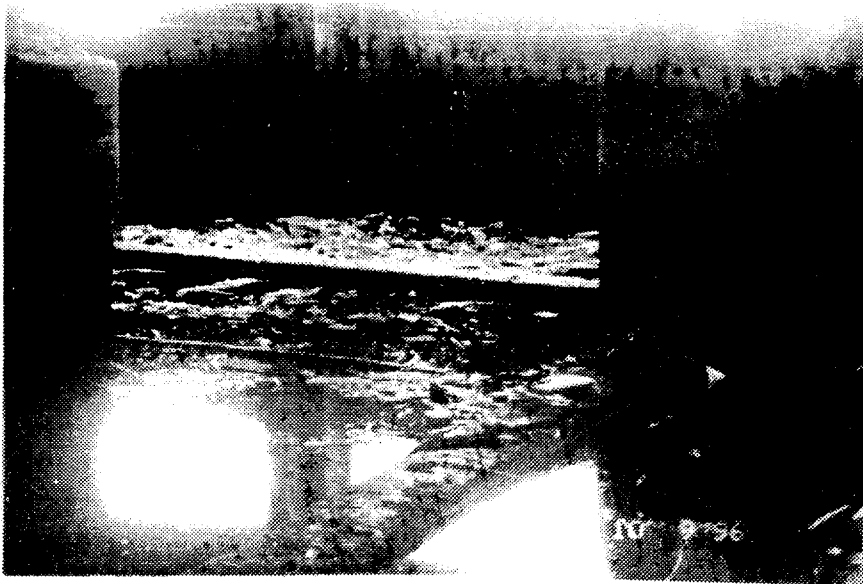
FLOATING TRASH, ACCUMULATED ON PIERS 15 AND 16
