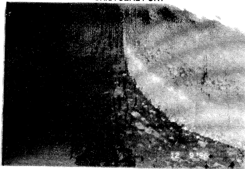
BIOFAULING IN THE PILASTERS OF PIERS (INDICATOR OF WATER QUALITY)
